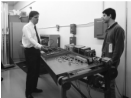
PEAC's Mark Stephens (left) and Doni Nastasi talk about fine-tuning the PLC project's test setup. The PLC (shown mounted at the top of the control board) is the brains of this simulated textile/paper production process.
